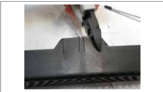
Cut holes to allow cable access
